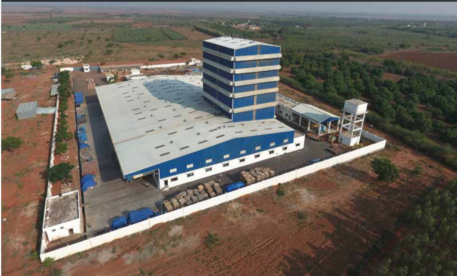
Aerial view of Shrimp feed factory—Pinnae Feeds Limited (since amalgamated with the Company)
